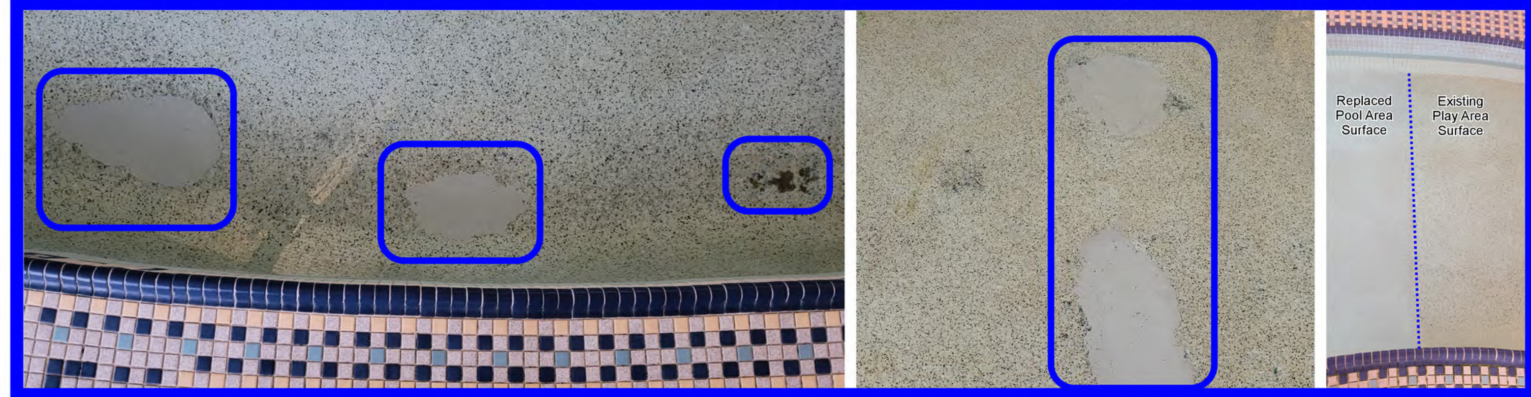
Water Play Structure Area Aggregate Flooring Replacement
