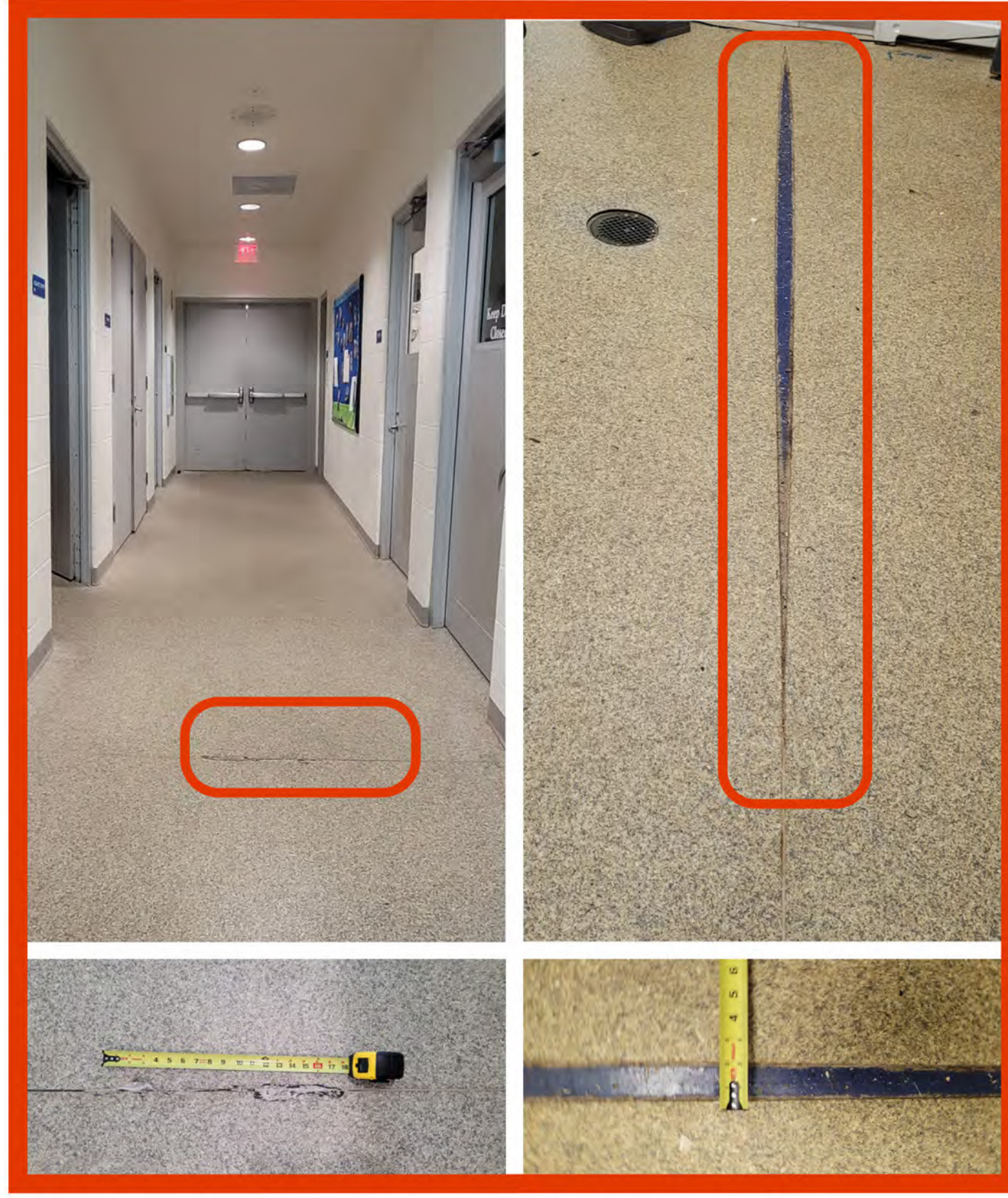
Aquatics Office Area and Party Room Flooring Replacement
