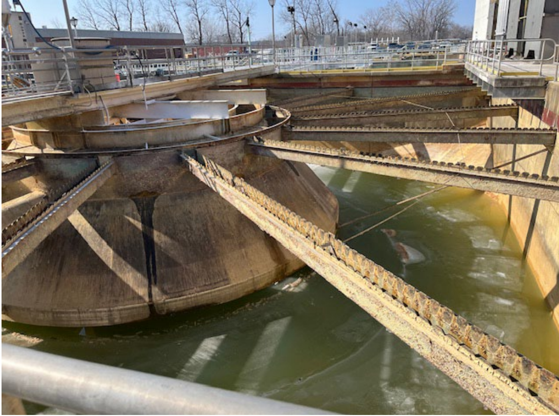
Primary Clarifier #:2: Starting demo process
