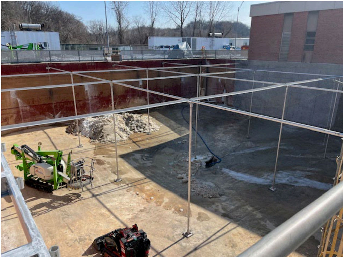
Secondary Clarifier #1: Starting baffles
