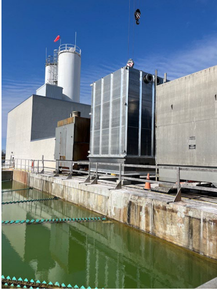
New Aerator #3 set
