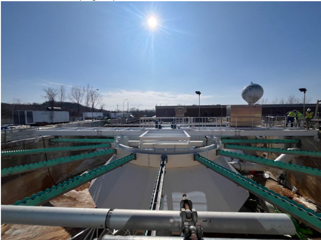
Primary Clarifier #1: Almost completed
