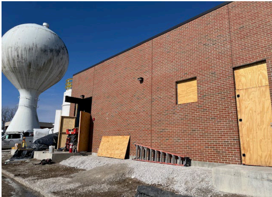
New Chemical Building: Working on electrical
