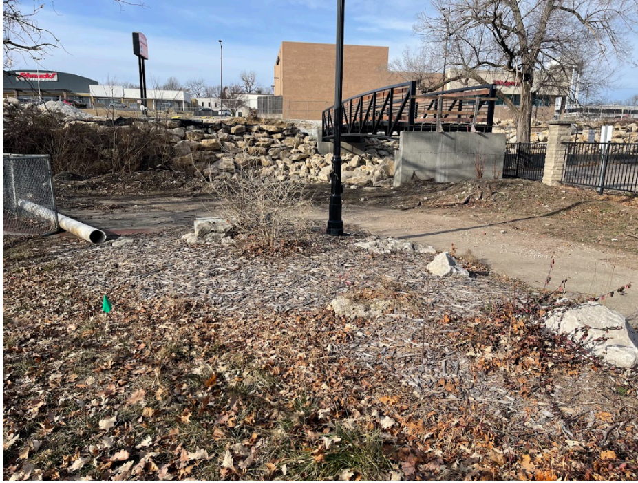
Photo 1: Approximate installation location.
