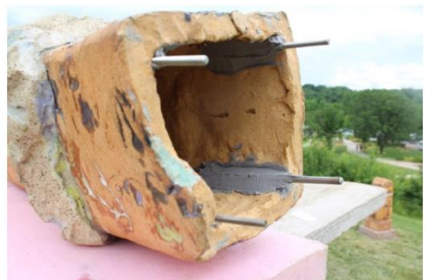
Example of repairs in progress for column 12
