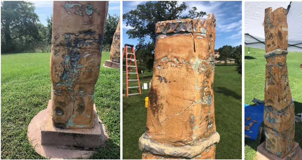
Column 11 repairs in progress
