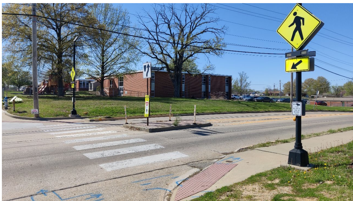
Photograph 10: N Garth Ave & Parkade Blvd (RRFB)
