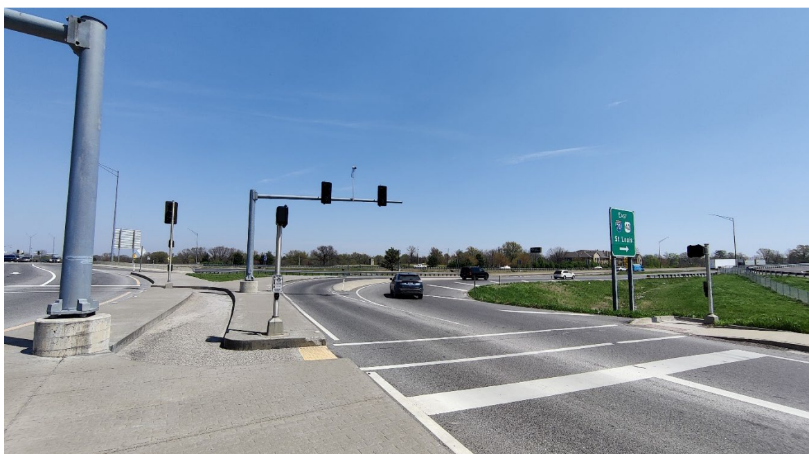
Photograph 16: Stadium Blvd DDI at I-70
