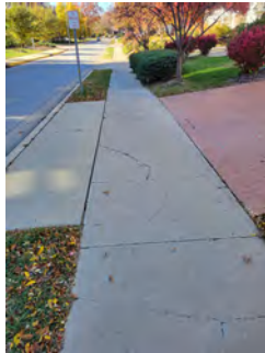
#2: REMOVE & RECONSTRUCT SIDEWALK PANELS (28'X5').
