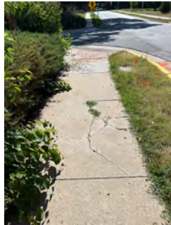
#4: REMOVE & RECONSTRUCT SIDEWALK PANELS (5'X5').
