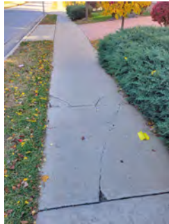
#3: REMOVE & RECONSTRUCT SIDEWALK PANELS (10'X5').
