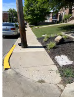
#2: REMOVE & RECONSTRUCT SIDEWALK PANELS TO WIDEN AROUND UTILITY POLE (15'X6').
