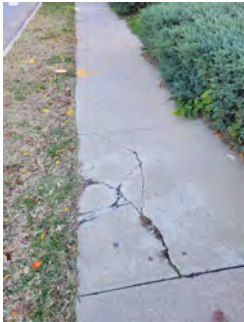
#1: REMOVE & RECONSTRUCT SIDEWALK PANELS (11'X5').
