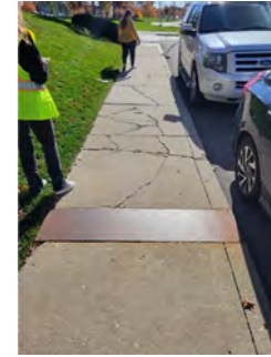
#7: REMOVE & RECONSTRUCT SIDEWALK PANELS (35'X5').
