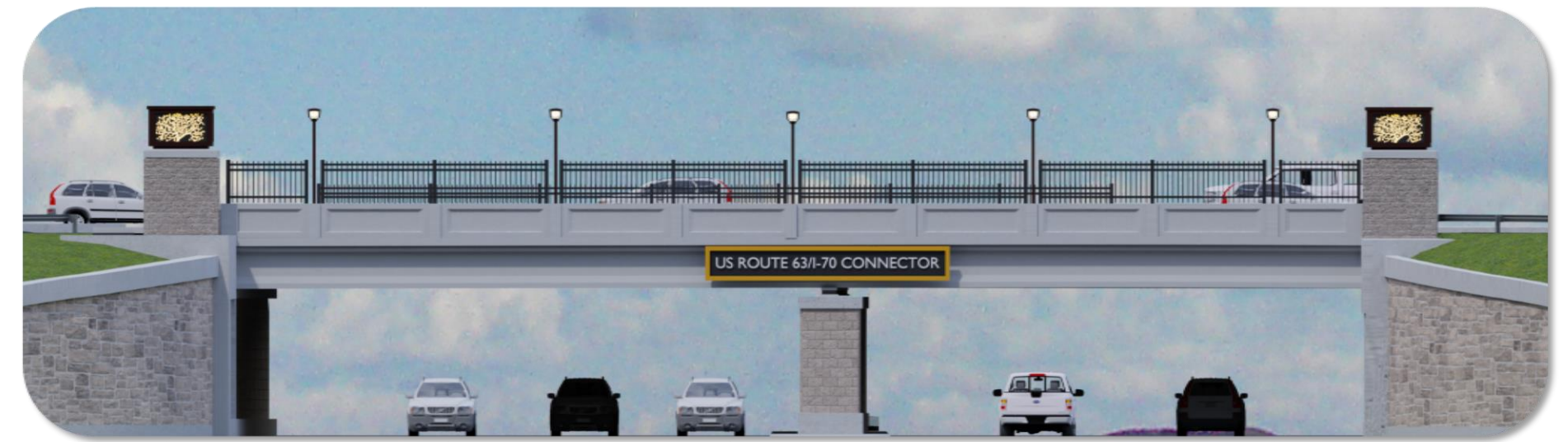
End piers terminate the bridge façade, fencing and bridge
