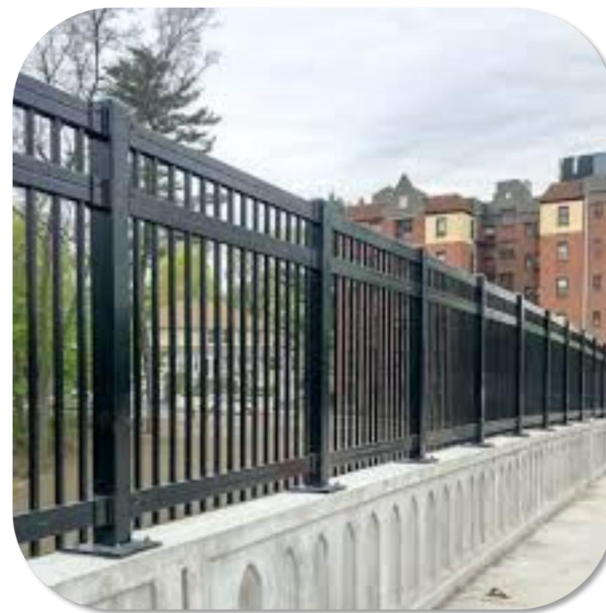
Ornamental metal fence on bridge barrier
