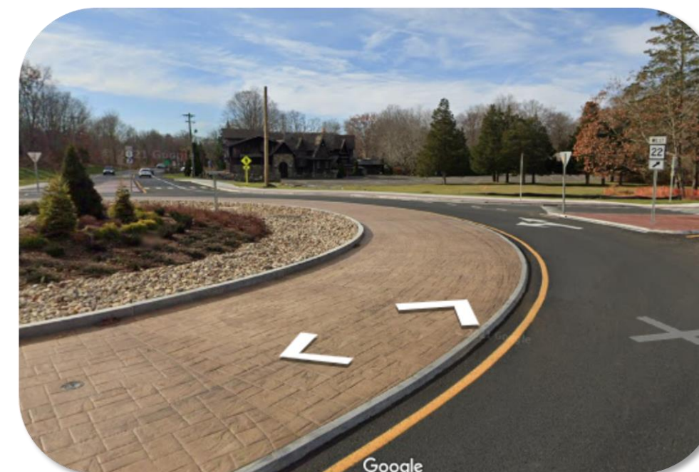
Example images for stamped color concrete truck apron
