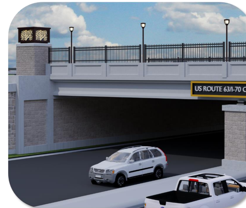
Example of ashlar formliner patterns and curved retaining walls
