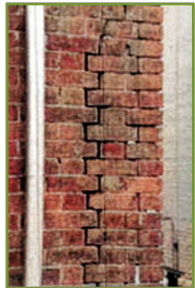
Improper drainage has caused failure in the corner of this historic brick building. Proper guttering and water diversion systems should be well maintained throughout the historic district.
