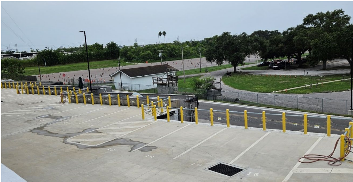
Figure 20: Back-In Parking Areas for Customers, City of Tampa “Z-Wall” Recycling Center
