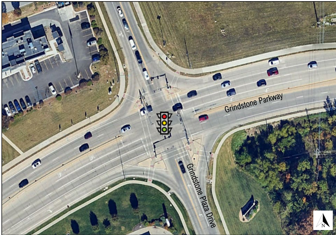
Figure 3: Aerial View of the Grindstone Parkway and Grindstone Plaza Drive Intersection
