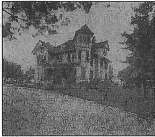
Constructed in 1883, the 20 room house, lake, and depot known as "Windemere" would feature a ballroom, billiard room, and smoking den. Its destruction by fire in 1913 led the City of Columbia to establish a professional fire department.
