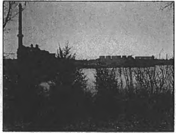
Built by Elawson More, the lake that bears his name is still visible on the City Power Plant property.
