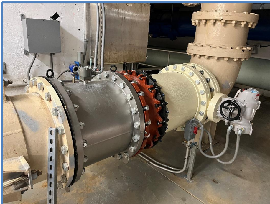
Figure 1 – New flow meter and valve for backwash line
