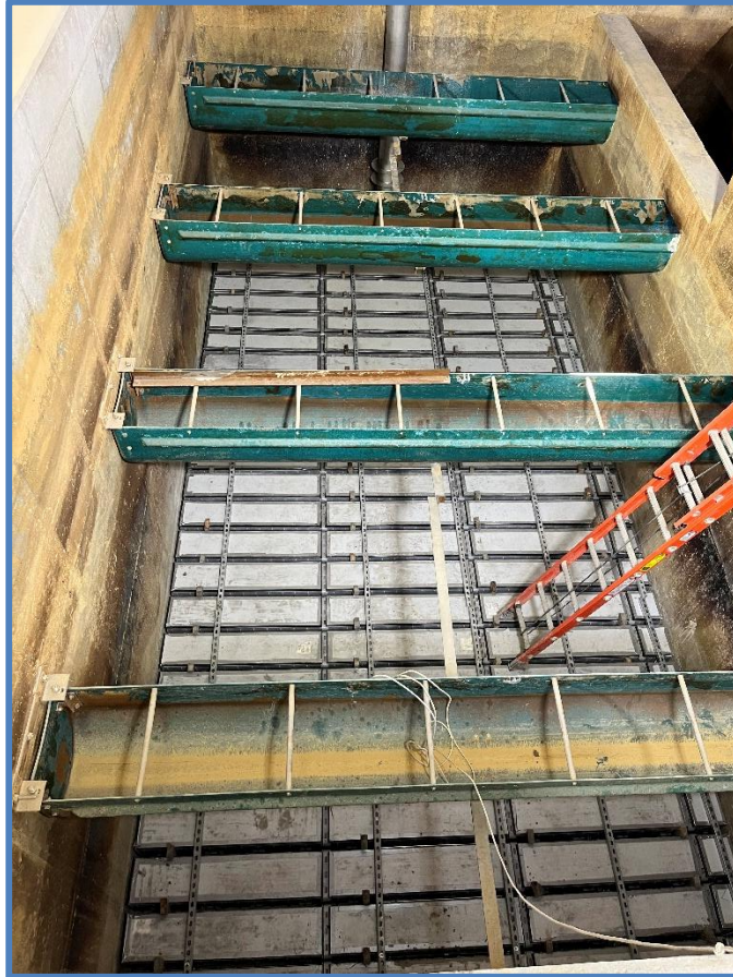
Figure 4 – Filters 7 & 8 installed (pre-grout)
