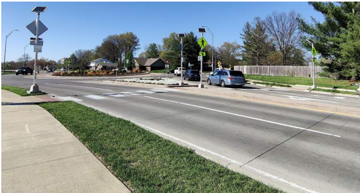
Photograph 7: Forum Blvd & Green Meadows (RRFB at Roundabout)
