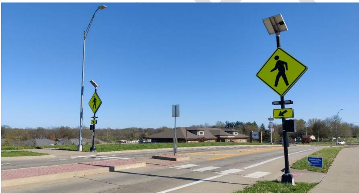
Photograph 8: Scott Blvd South of Abbington Terrace (RRFB)
