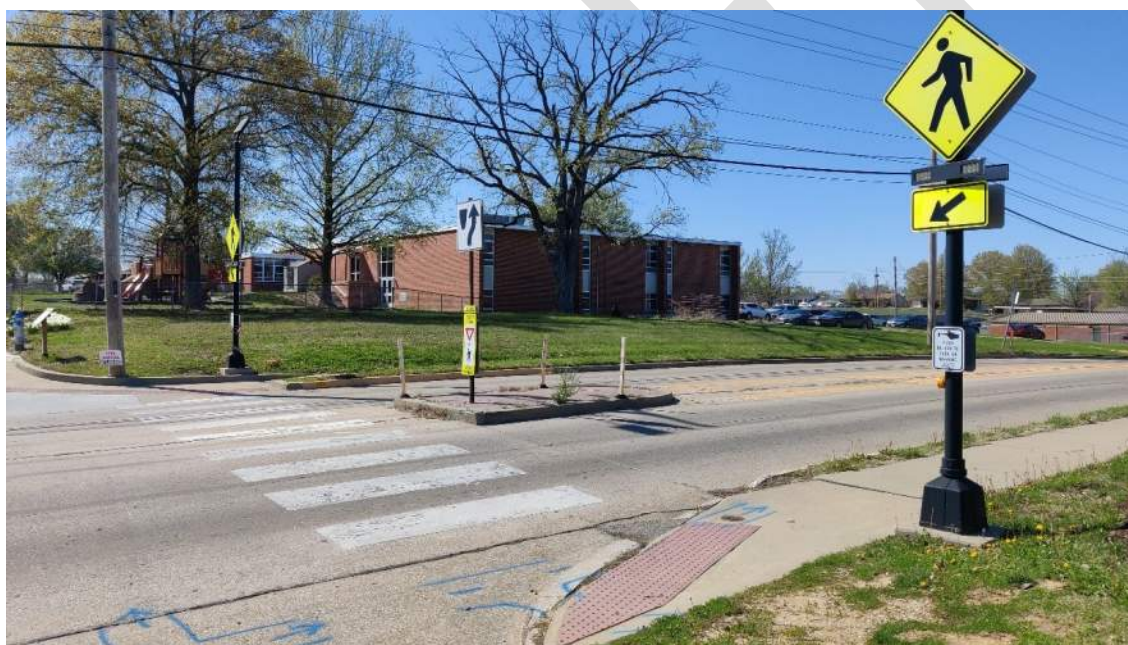
Photograph 10: N Garth Ave & Parkade Blvd (RRFB)
