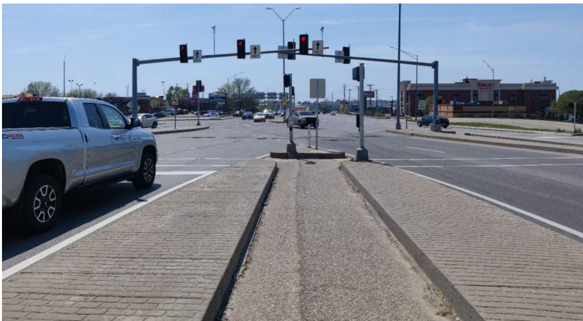
Photograph 17: Stadium Blvd DDI at I-70 (Pedestrian Bridge)
