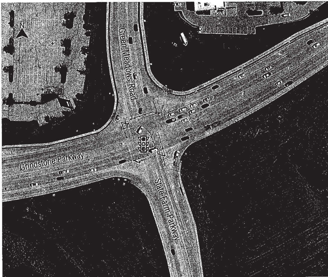
Figure 7: Aerial View of Grindstone Parkway and State Farm Parkway/Green Meadows Road
