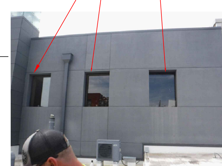
RI 12. WET-SEAL NORTH ELEVATION WINDOW SYSTEM.
