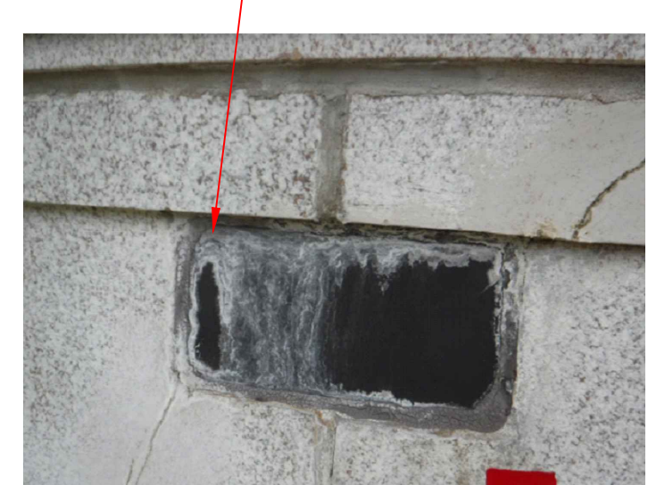
RI 13. SEAL ATTIC VENT COVERS.
