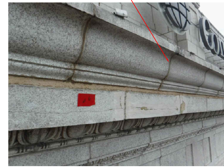
RI 4. REPLACE TC UNIT JOINT MORTAR/SEALANT AT 100-PERCENT OF THE TC UNIT SKYVIEW SURFACES AS INDICATED ON THE DRAWINGS.
