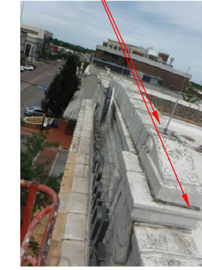
RI 4. REPLACE TC UNIT JOINT MORTAR/SEALANT AT 100-PERCENT OF THE TC UNIT SKYVIEW SURFACES AS INDICATED ON THE DRAWINGS.
