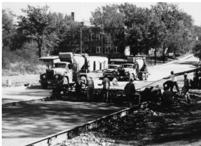
[Park Avenue Construction, Douglass HS, (1961) Tapp-Elbert, Wynna Faye, SHSMO. C4057-f010-021.]
