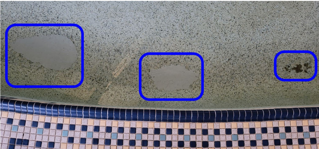
Water Play Structure Area Aggregate Flooring Replacement
