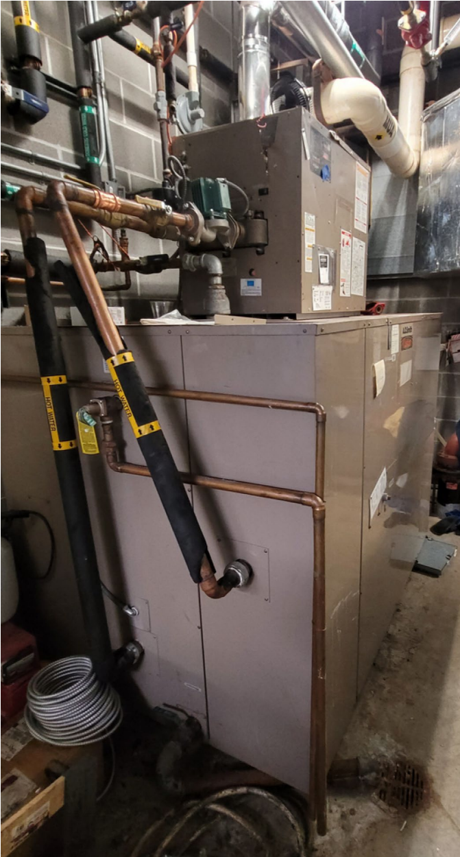
Domestic Hot Water Heater Replacement
