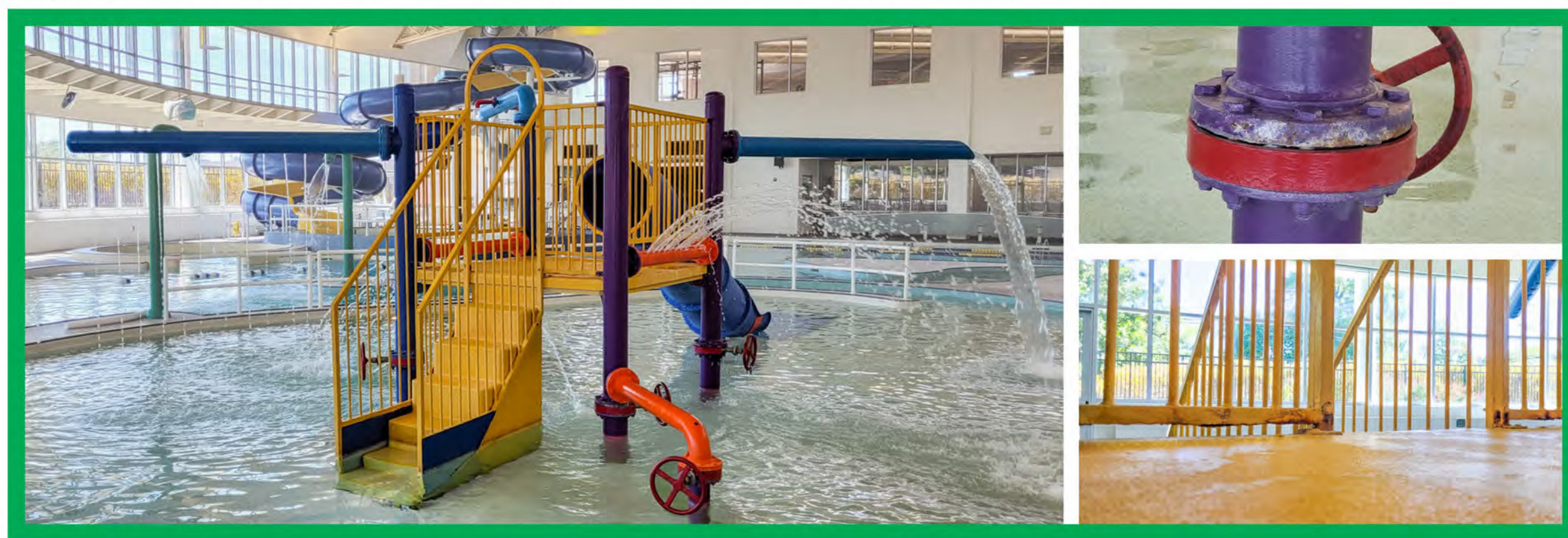
Water Play Structure Replacement
