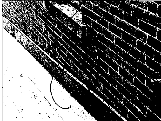
Surface-mounting wires on historic buildings in Enfield should be avoided.
