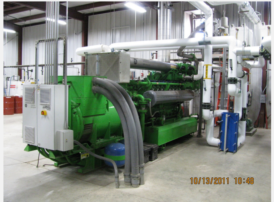
Landfill Gas Plant Engine – 1 MW
