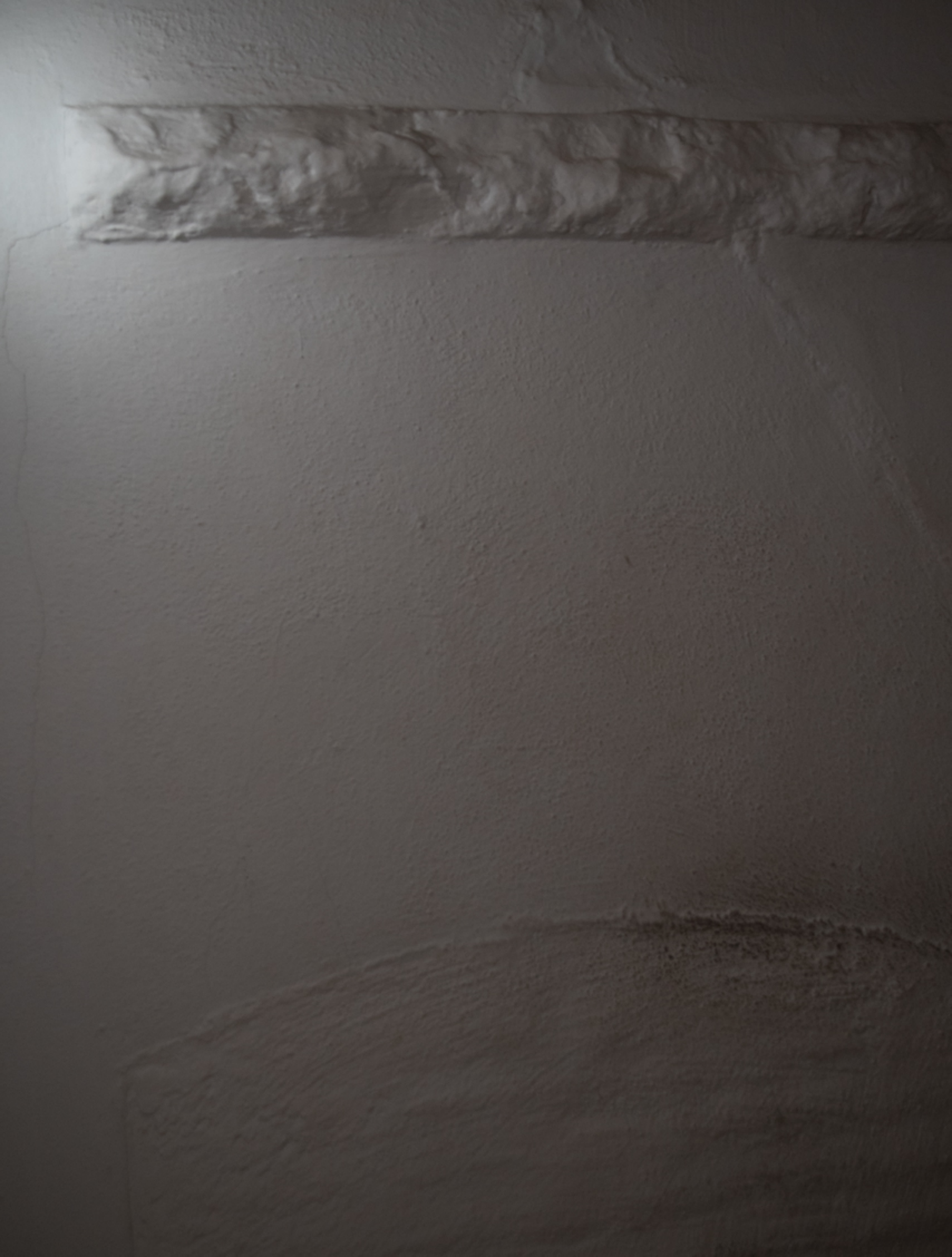
Enclosed Windows - Stone Sill (above) & Arched Lintel (below)
