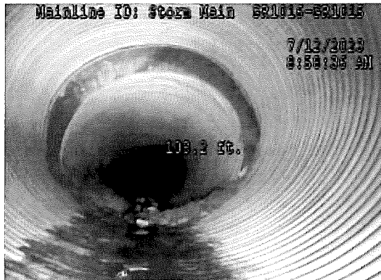
Joint Separation with soil intrusion into pipe. Location is approx. underneath sinkhole
