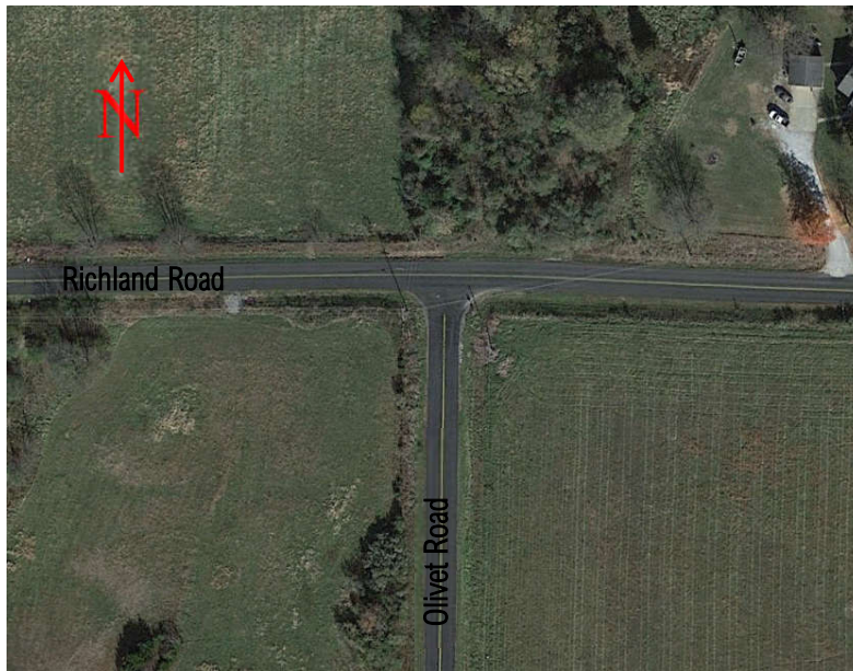
Figure 5: Aerial View of the Richland Road and Olivet Road Intersection
